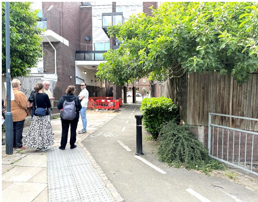
Residents on the walkabout considering the issues by James Stewart House underpass
