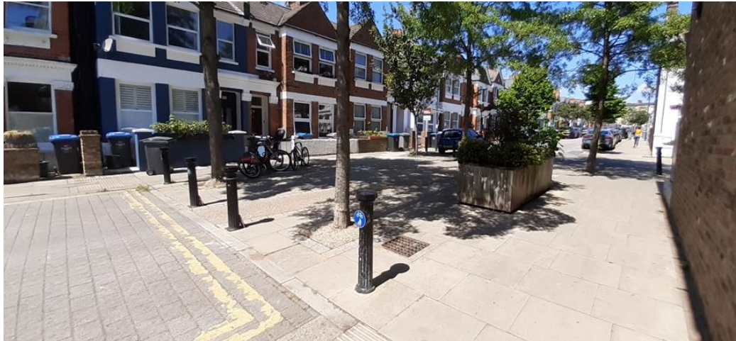
Existing modal filter on Tennyson Road, the other side of Willesden Lane
